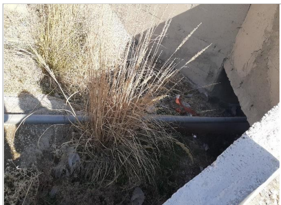
Figure-4.17: View of pipe passing through under Bypass Road
